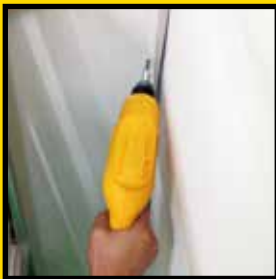
2 Driving Screws On Window Frame & Drill Holes In Wood Frame 10mm Rotary Drill STD5510
